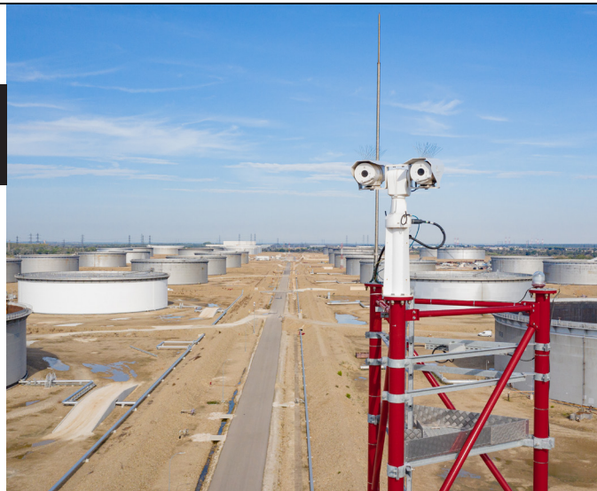
Three thermal camera systems, installed on 30-meter poles, scan the entire 160-hectare SPSE site on a 24/7 basis.
