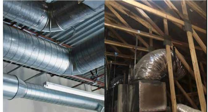
*When duct work is improperly installed or develops air leaks, HVAC systems will run inefficiently.*
