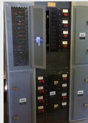
24-inch IR window installed at SLAC
